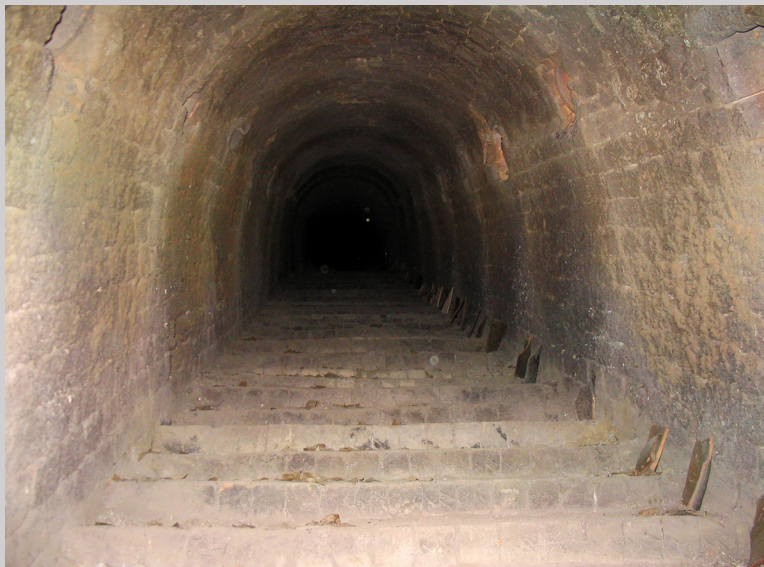
Figure 5.8g The sloped floor inside the kiln is stepped so that pieces can be stacked on a stable, horizontal surface. It takes six months to fill with work, so this dragon only fires up twice a year in Tianbao, China (photograph by Carol Ventura, 2004).
