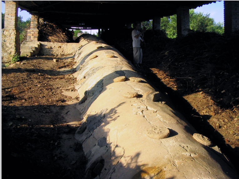
Figure 5.8f This dragon kiln has side entrances for loading firewood and port holes (plugged in the photo) on the roof for stoking. Most of the kiln is underground (to conserve heat); only the arched roof is left uncovered in Tianbao, China (photograph by Carol Ventura, 2004).
