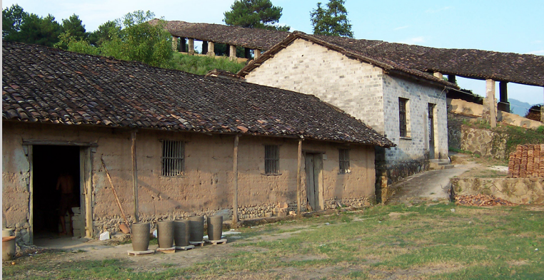
Figure 5.8d Pots dry in front of the pottery workshop. A tile roof protects the 160 ft / 48.77 m long wood-fired dragon kiln that runs up the hill behind the workshop in Tianbao, China (photograph by Patty Haag, 2004).
