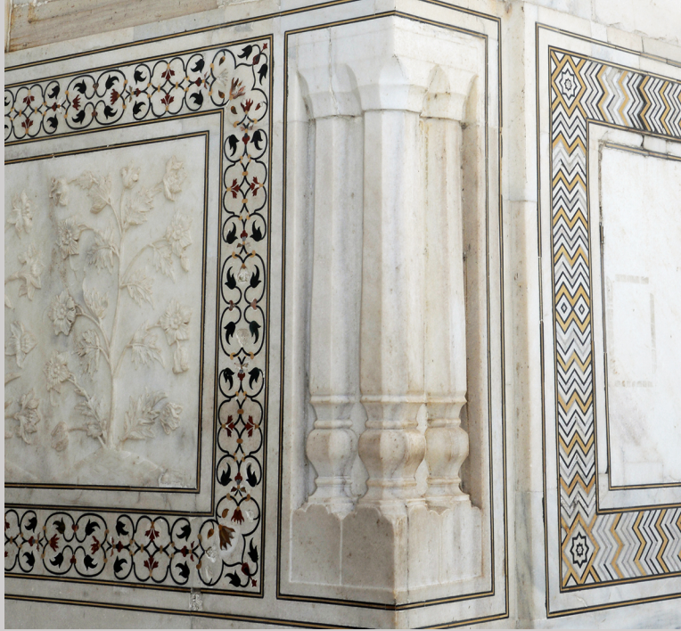
Figure 5.39a Stone inlaid into the marble walls of the Taj Mahal, Agra, India (photograph by Carol Ventura, 2016).
